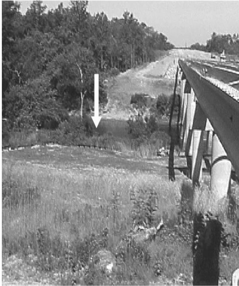
Figure 4. Photograph of the deeply incised Cape Fear River during construction of the Fayetteville Outer Loop.
