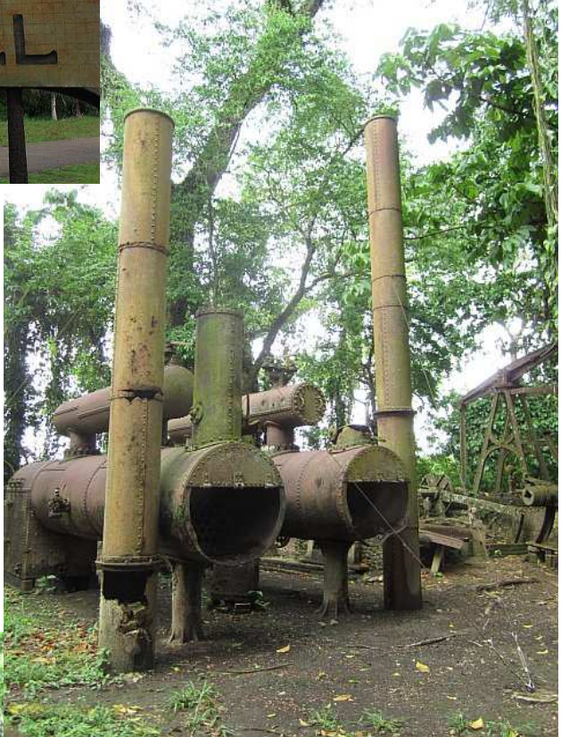
Figure 9. Sugar Mill machinery at Serpon Sugar Mill
