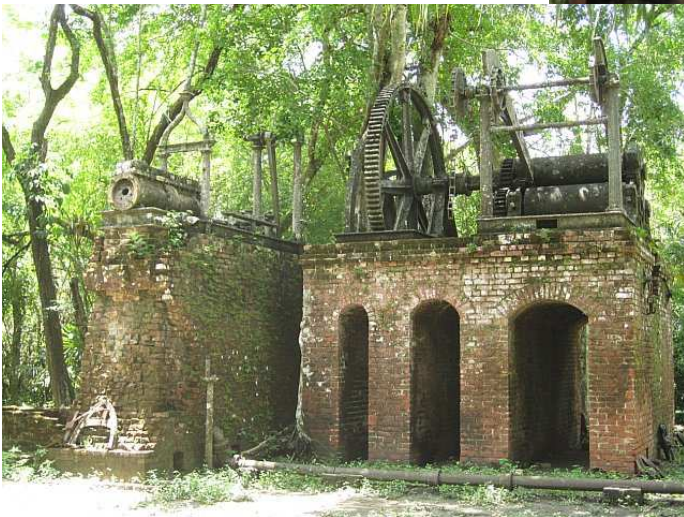
Figure 15. Photo of some Machinery at the Lamanai Sugar Mill
