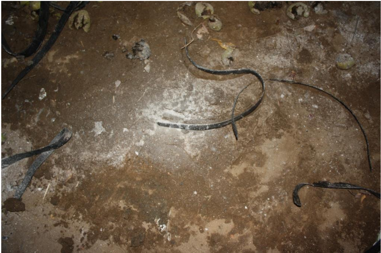
Fig.4 Dirt Floor with Belts
