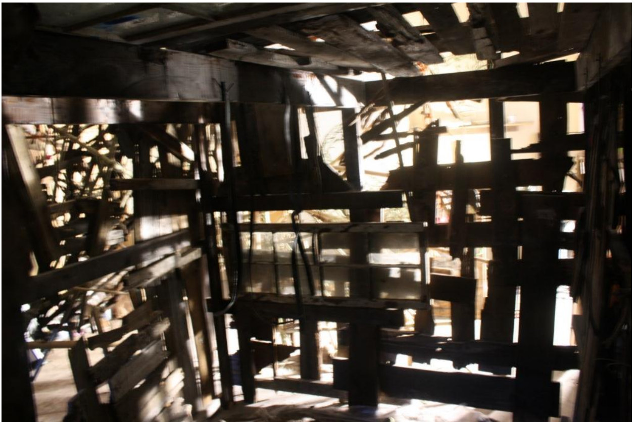
Fig.5 Interior of Wooden Structure
