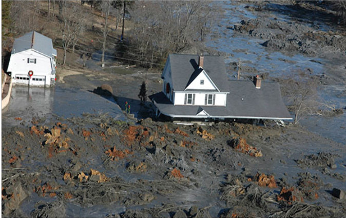
Figure 3 – Fifteen homes were destroyed as a result of the collapse of an earthen retaining wall at the Kingston Plant (Dewan, n.p.)
