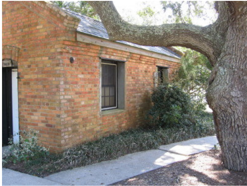
Figure 9: The Oilhouse at Old Baldy, plans are to turn this building into exhibit space that will focus on the technological history of the site.
