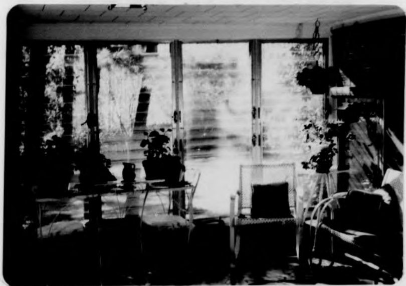
Figure 5.--Type of Enclosure--Jalousie. Two Views of One of the Most Used Glassed Porches.
