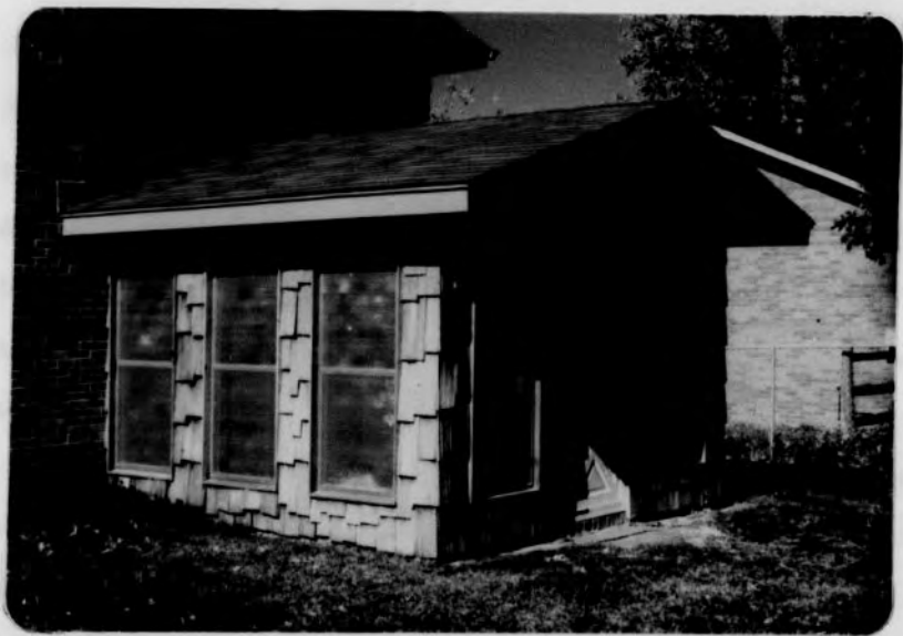
Figure 4.--Type of Enclosure--Sliding Storm Window. Two Views of a Glassed Porch that was Once a Sunken Patio.
