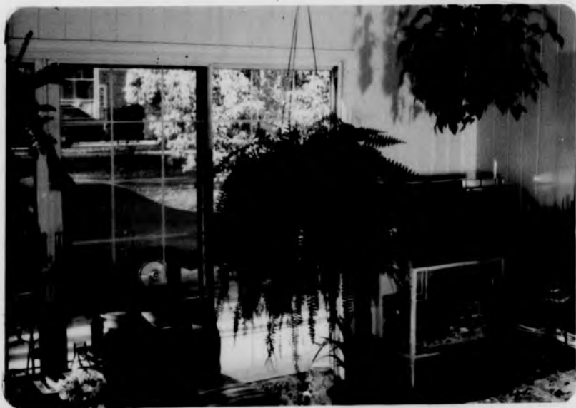
Figure 8.--Type of Enclosure--Tinted Sliding Glass Door with Muntins. Two Views of the Most Used of all Porches in the Study.
