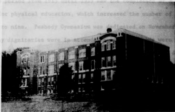
Figure 14. Peabody Gymnasium During Construction, 1915
