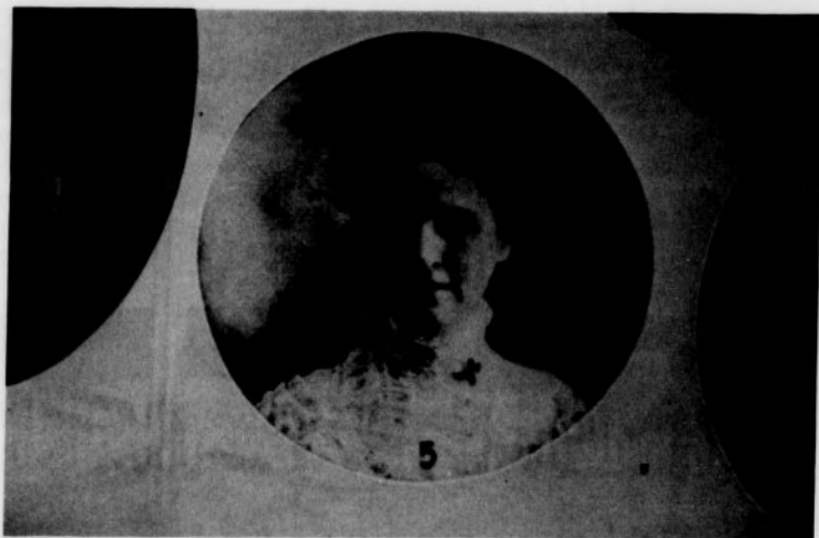
Figure 5. Ada Wolfe, 1901 building
