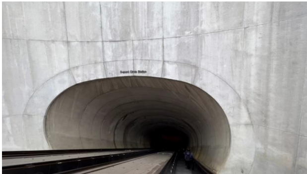
Figure 3. Escalator into Dupont Circle station 8
