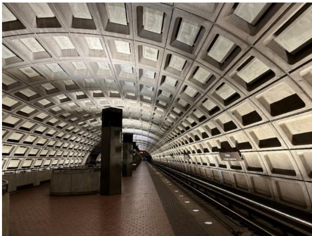
Figure 5. Rosslyn station's indoor pylons 11
