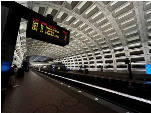
Figure 4. Clarendon station platform with hexagonal floor tiles and waffle ceiling design. 10
