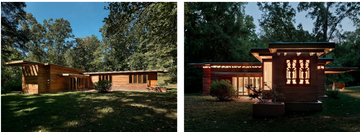
Figure 30. View of the Backyard and Patio of the Pope-Leighey House (Burk, 2013)
