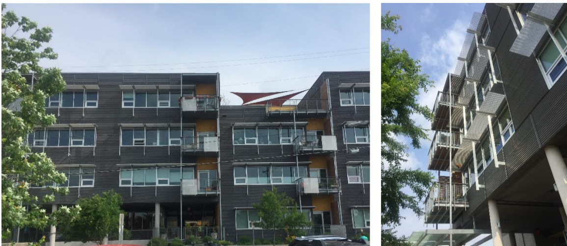
Figure 26. Front Façade of Durham Central Park Cohousing Community
