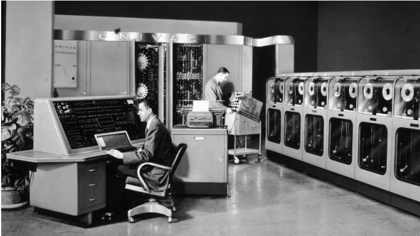
The commercial computer UNIVAC I, designed by John Mauchly and J. Presper Eckert, the inventors of ENIAC [1951]. (2013, June 23).
