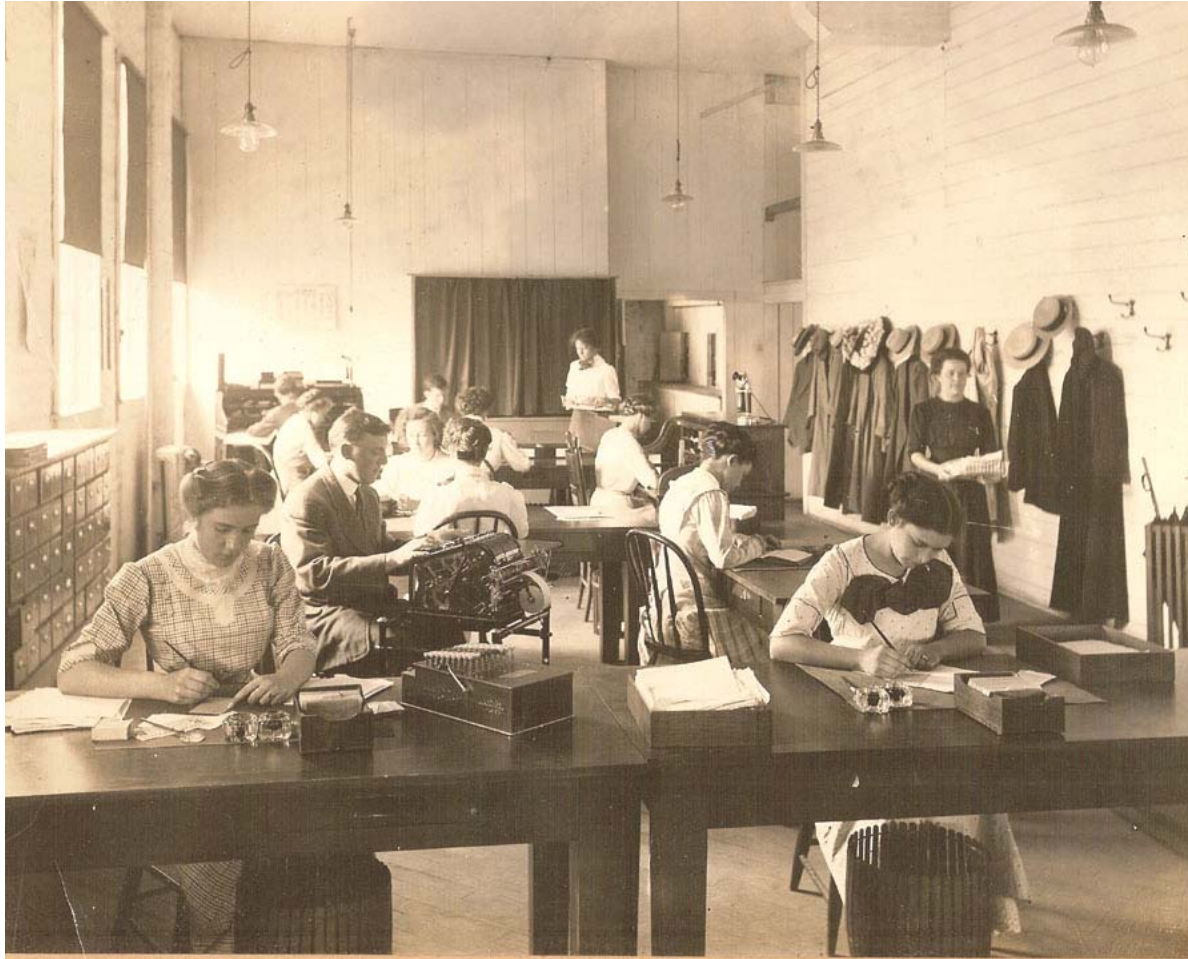
Ladd & Son. (n.d.). Office of Giant Clothes Store, Muskegon, MI [There is a Comptometer Model A calculating machine (sold 1904-06) in front of the woman on the left. The man behind her is working on a Burroughs Class 1 Adding Machine.]
