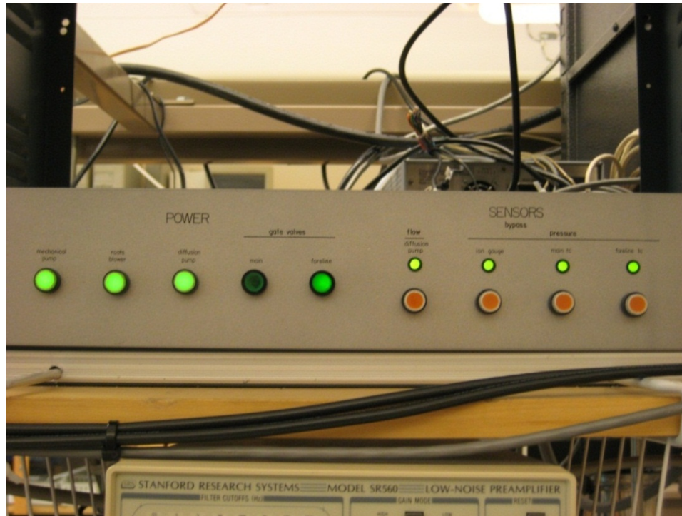
Figure 17. Interlock system. The five buttons on the left turn on/off the pumps and open/close the gate valves on the chamber. The left four buttons are tied to the pressure and water flow sensors so that if there was a spike in pressure or the water cooling the diffusion pump stopped, which could damage the pumps, the entire system will shut off.
