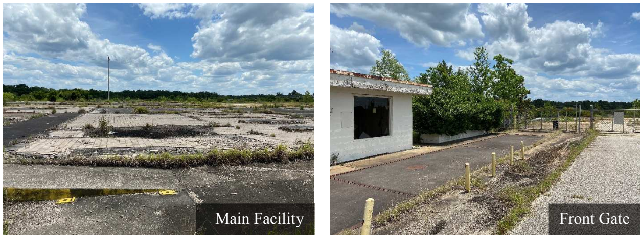
Figure 22. Defunct Syngenta Facility in Lemoyne, Alabama
