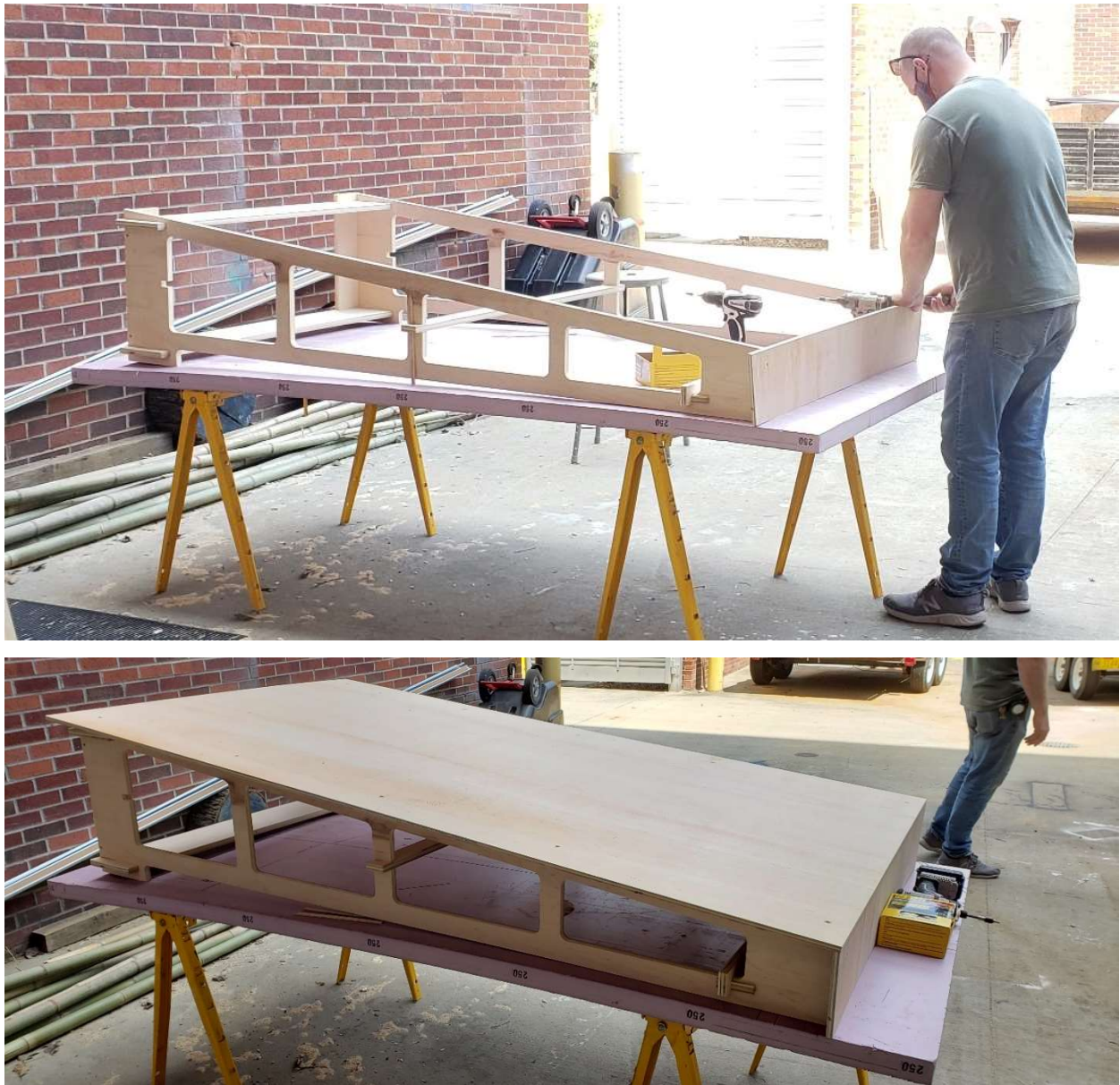
Figure 97. Gallery wall construction stages
