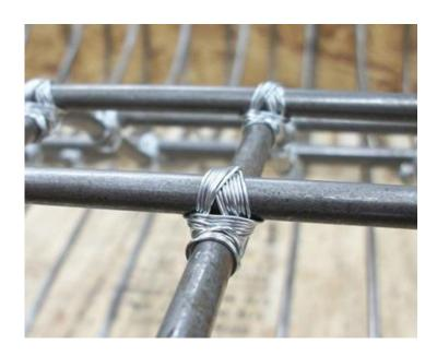
Figure 14. Lash Knot Detail
