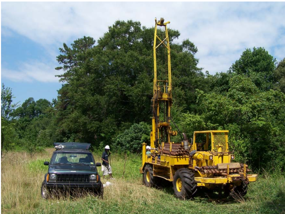
Figure 4.2 – Torque testing – NCDOT drill rig
