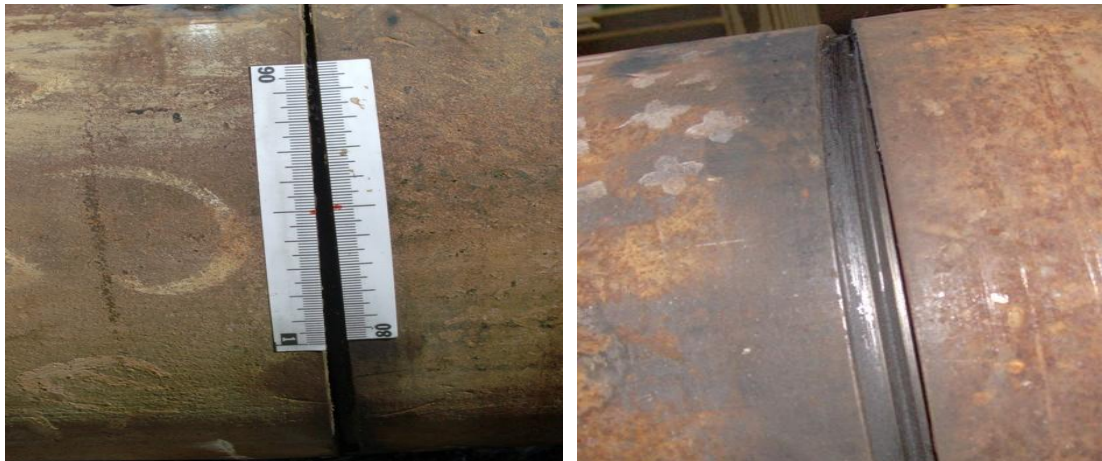
Figure 5.32: Failure mode of one of the tested micropile
