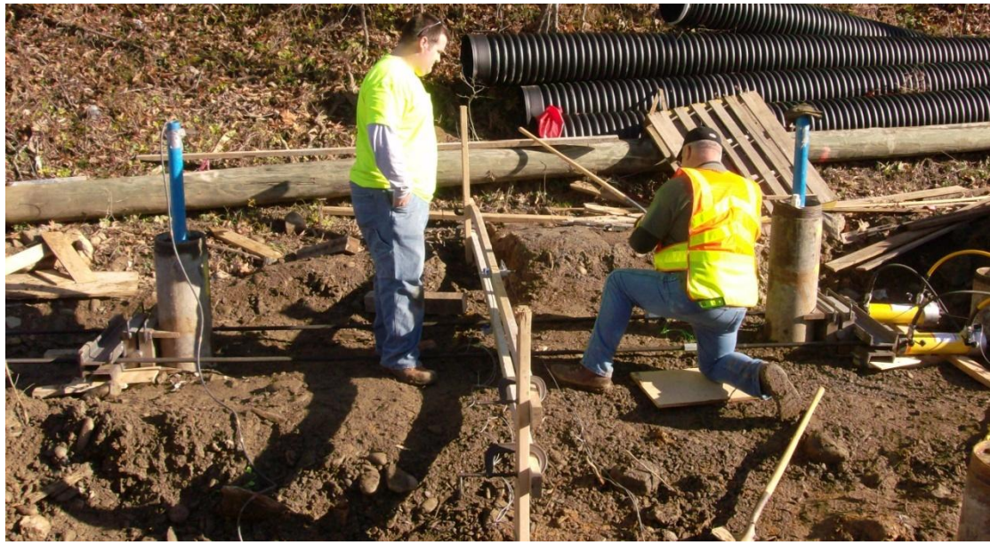
Figure 4.5: Load testing frame
