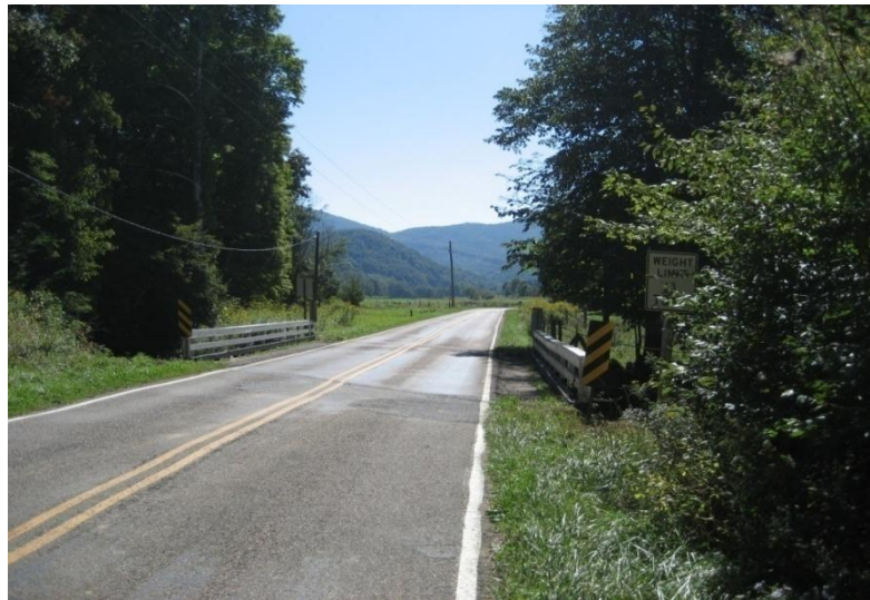
Figure 3.2: Photo of the bridge alignment along the road
