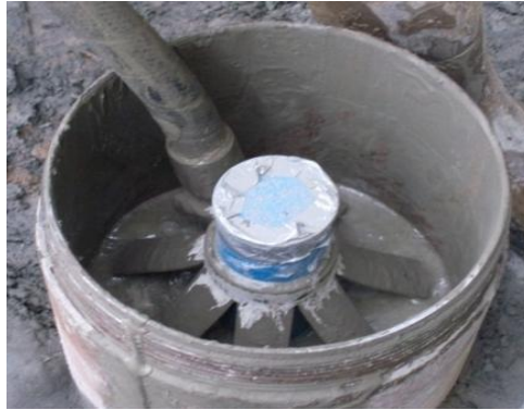
Figure 4.12: Photograph of cast micropile with Instrumentation cage.
