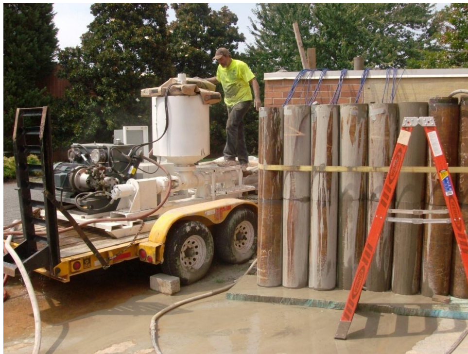
Figure 5.3: Grouting micropile specimens
