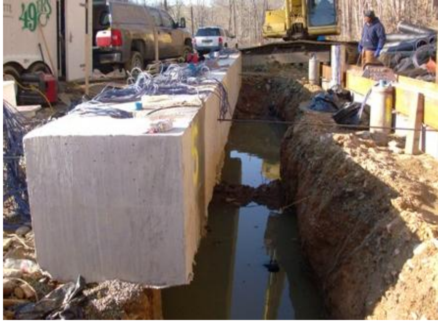
Figure 4.40: Pile group testing in progress.
