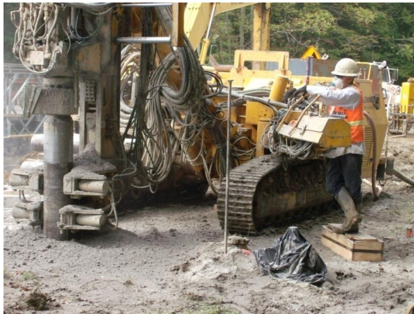
Figure 2.4: Typical micropile construction
