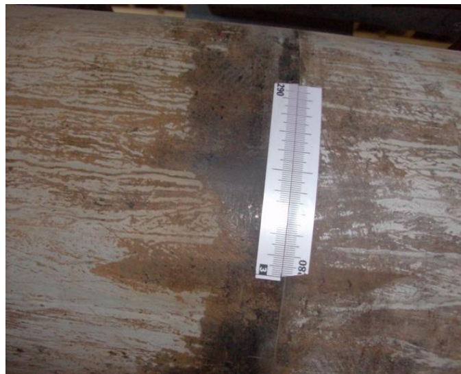
Figure 5.6: Measuring casing twist using scale tape
