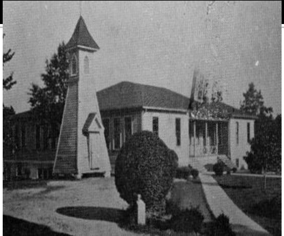
The original (1910) Dining Hall and Bell Tower of the National Religious Training School
