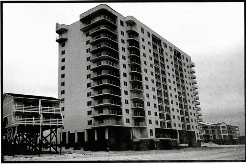
Figure 6. This large condominium was constructed on deeply driven concrete pilings which allowed it to withstand Ivan's storm surge, storm waves, and the loss of beach sand from in front of and beneath the building. Image from November 2004.
