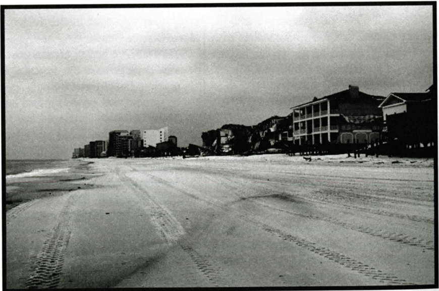
Figure 5. A large section of the coastline at Orange Beach has been flattened by Hurricane Ivan's storm surge and erosive storm waves. This was the state of the shoreline and beach on November 2004. View looking west.
