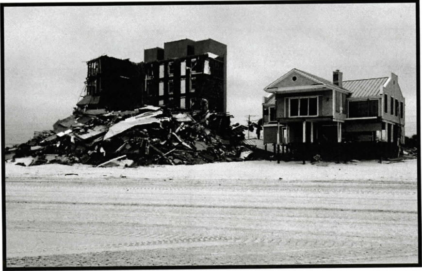
Figure 4. This photograph of the two structures shown in Figures 3a and 3b reveals that considerable beach sand has been removed by Hurricane Ivan's storm surge and erosive storm waves. The painted wooden stilts indicate the former elevation of beach sand beneath the house. The unpainted portion of the stilts at the front of the house is approximately 2.4 m above the ground surface. The adjacent small condominium was constructed on an unsupported concrete slab that was undermined during the course of the storm by the elevated storm surge and storm waves. Image from November 2004.
