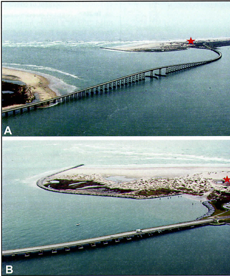
Figure 3. Oblique aerial photographs show the Oregon Inlet bridge that was built in 1962-63. Panel A is looking SW from Pamlico Sound with Bodie Island on the left and Pea Island on the right. Panel B is a close-up of the south end of the bridge and shows the terminal groin and reinforced rock revetment (built in 1989-91) around the base of the bridge. Red stars show the location of the abandoned US Coast Guard Station. Both photographs were taken on 11-16-2009 by the Pea Island National Wildlife Refuge.
