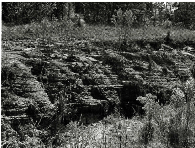
Figure 3. Channel margin IHS deposits at Middleground. Note erosionally resistant layers that are dominated by clay.
