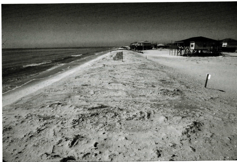
Figure 1. Facing west along the western low-lying developed portion of the island. The image was taken November 2000 following the construction of a berm designed to reestablish a beach and reduce flooding across this portion of the island. Approximately 229,366 cubic meters of sand was added to this portion of the beach (Henderson, 2005a). This was the largest beach renourishment project that I have witnessed in my many years of photographing various portions of the island. It was eroded away in only a few years.
