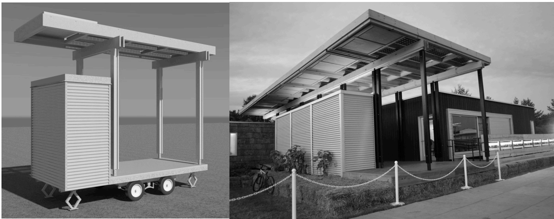
Figure 3. Individual OM rendering (left) and Solar Homestead photo on National Mall (right). Seven OMs combine to form the Great Porch and bifacial PV canopy, with three Kaco central inverters located in OM closets.
