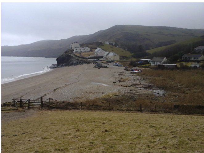
Fig. 3. Washover gravel in the marsh behind the Hallsands barrier in April 2013.
